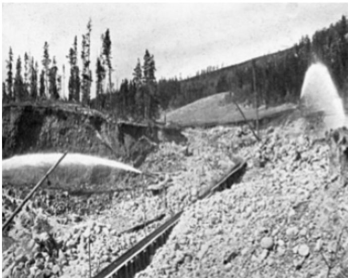
Hydraulic mining at the Snow Storm Mine. Note the sluice running through the middle of the site
